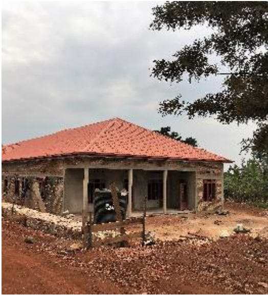
Figure 2.1: New building for pineapple drying under construction in 2019
