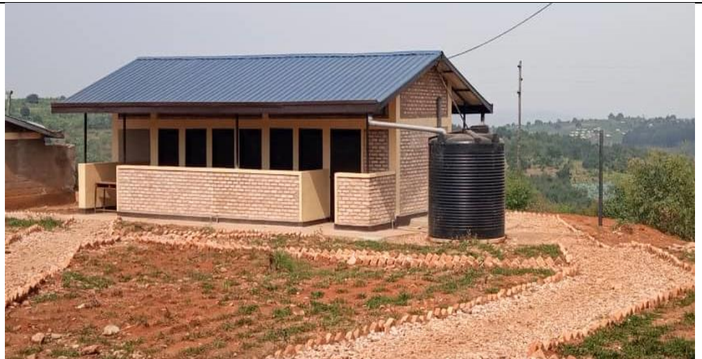
Block of 12 latrines constructed
