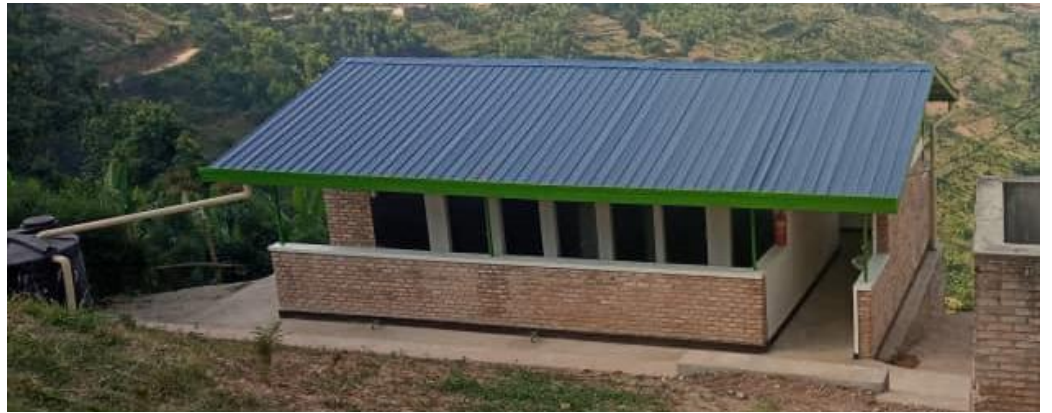
Block of 12 latrines
