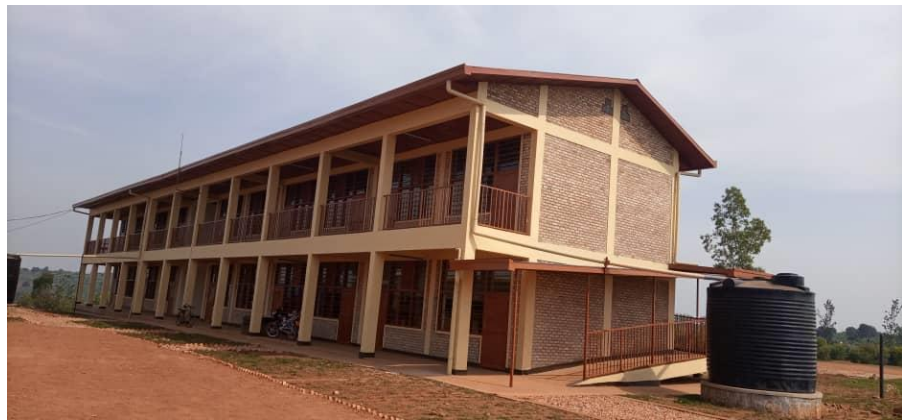
Block of 10 classrooms
