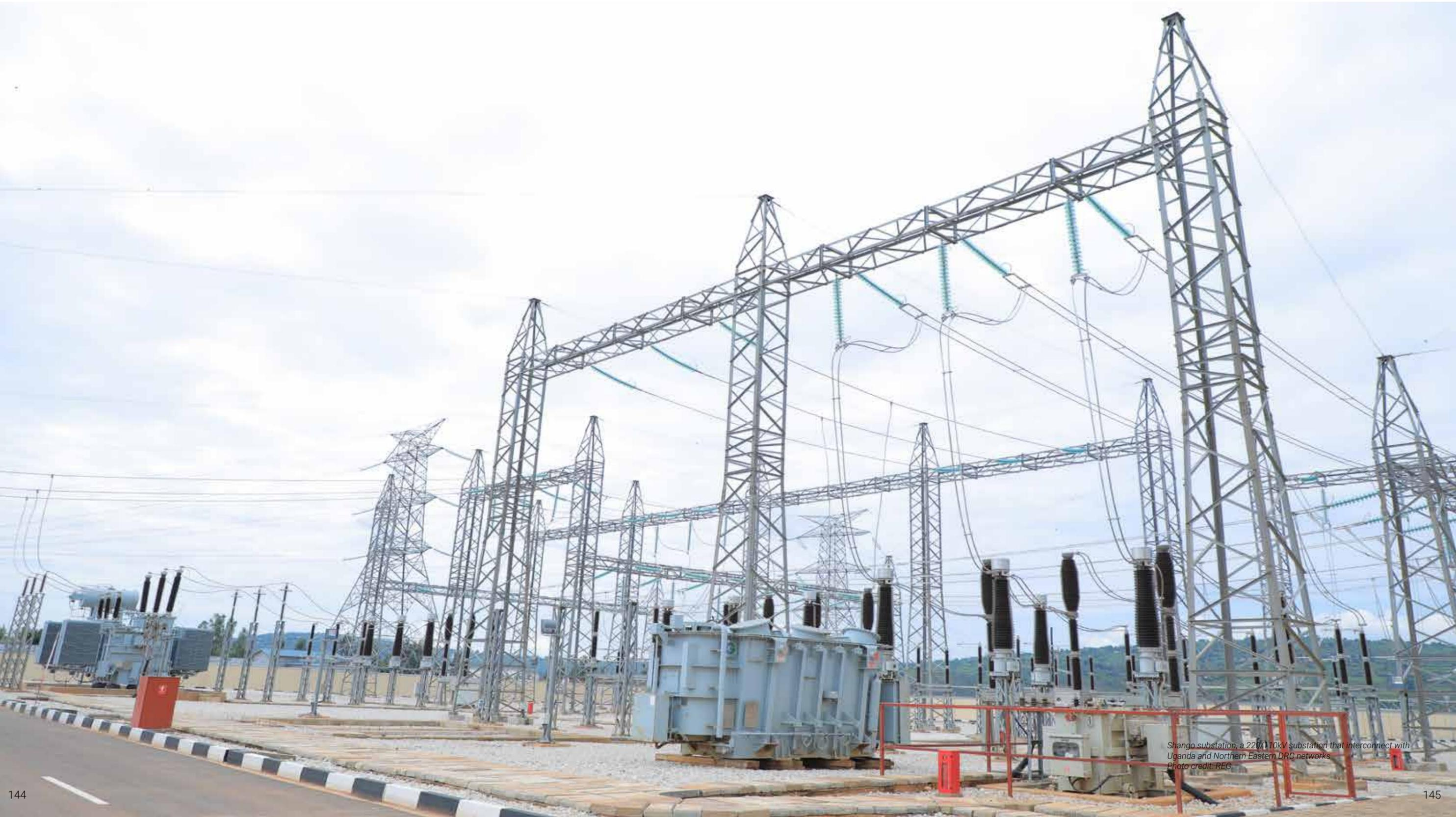
*Shango substation, a 220/110kV substation that interconnect with Uganda and Northern Eastern DRC networks
