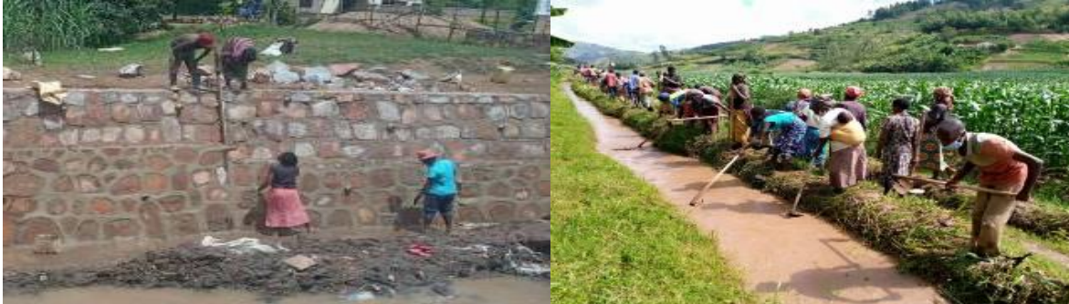
Photo 95: Rehabilitation of irrigation channels in Bishenyi marshland (left) and community work in Rufuka (right)
