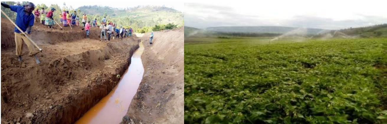
Photo 96: Deviation of Base river in Gashenyi sheme (left) and Irrigation in Nyagatare (right)
