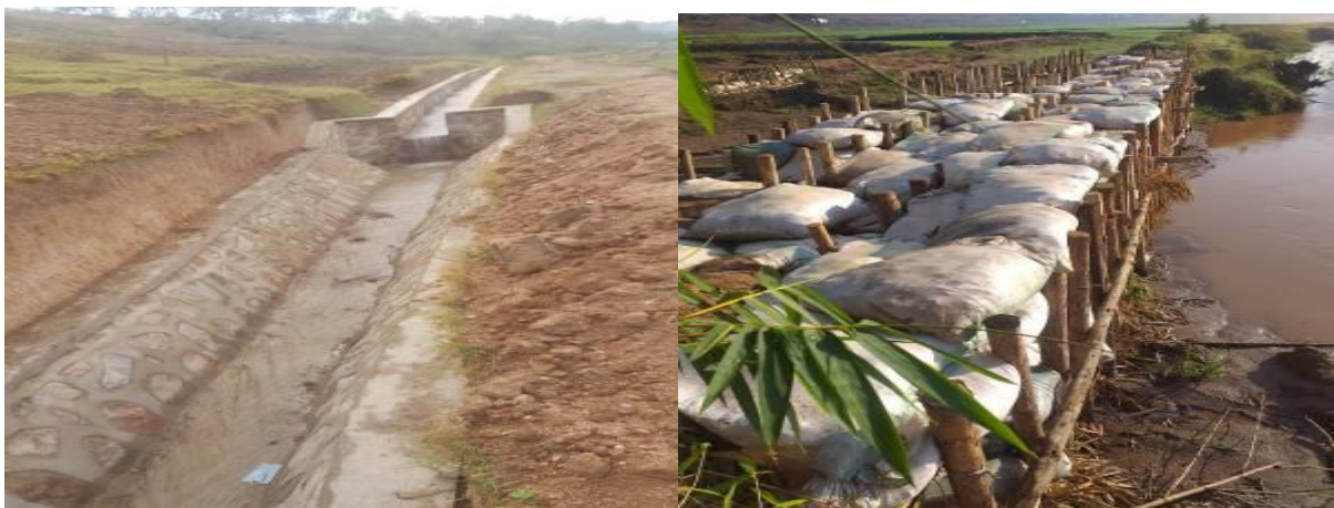
Photo 92: Repaired channel in Busogwe (left) and repaired dam in Jabana (right)
