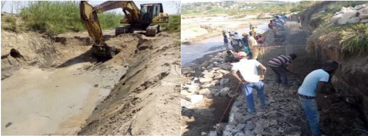
Photo 93: Excavation of Mukunguli River (left) and construction for gabions (right)
