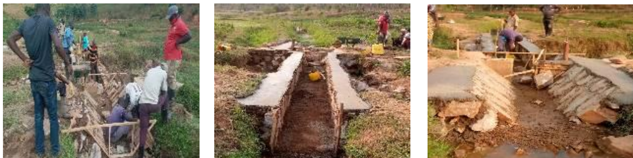
Photo 130. Practice of basic civil works in Ngoma 22
