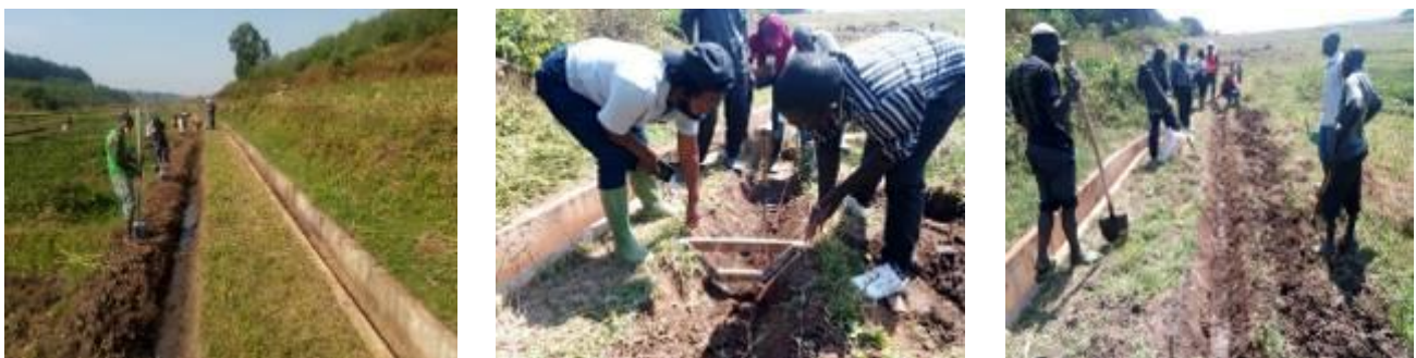
Photo 142. Creation of the Secondary canal in Cyimpima scheme
