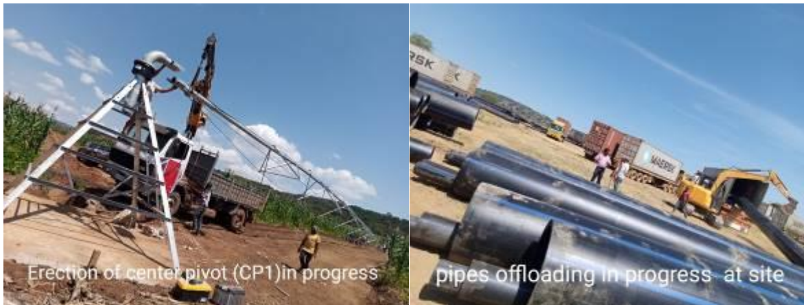
Photo 165. Erection of the center pivot and pipes offloading at Mpanga
