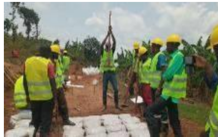
Photo 114. Compacting Do-nou Bags and illustration after the road is repaired in Ngiryi
