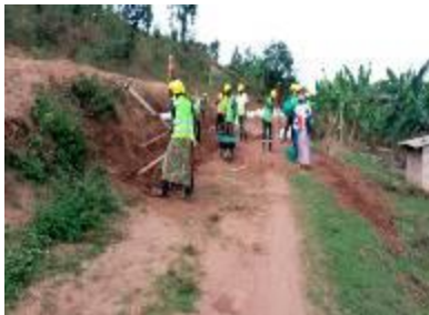
Photo 114. Compacting Do-nou Bags and illustration after the road is repaired in Ngiryi
