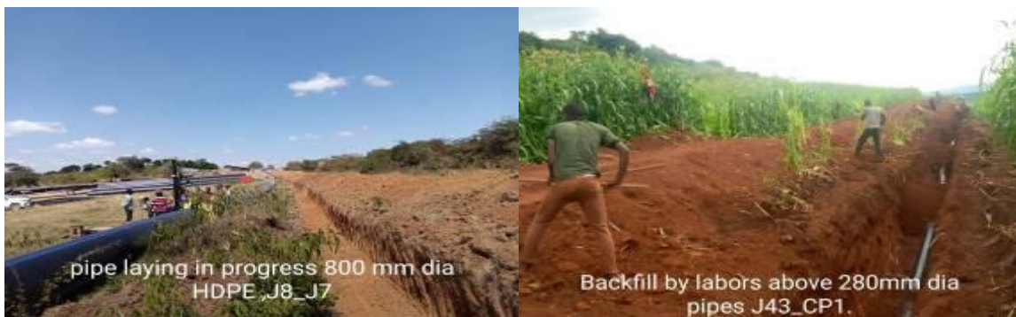
Photo 167. Pipes laying at Mahama 2
