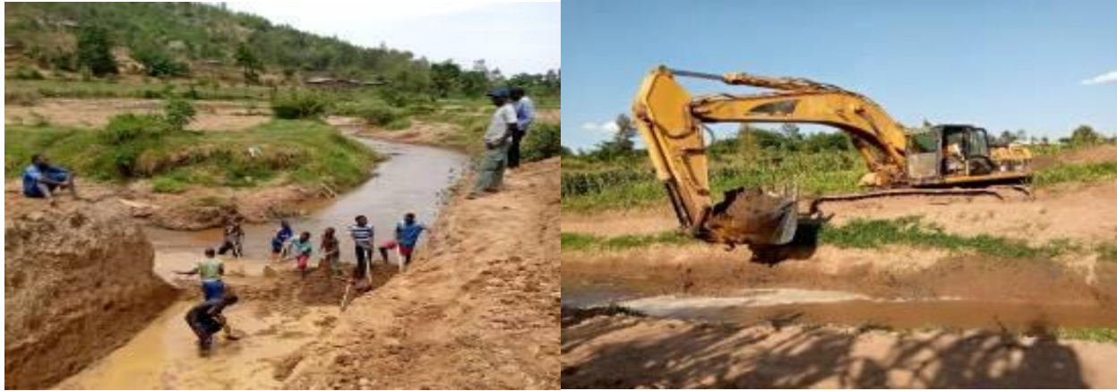
Photo 89: Temporary River deviation to allow the construction
