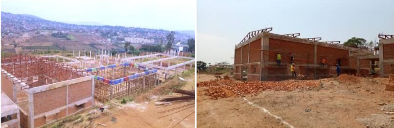
Photo 166. View of the Center of Excellence for Mechanization under construction
