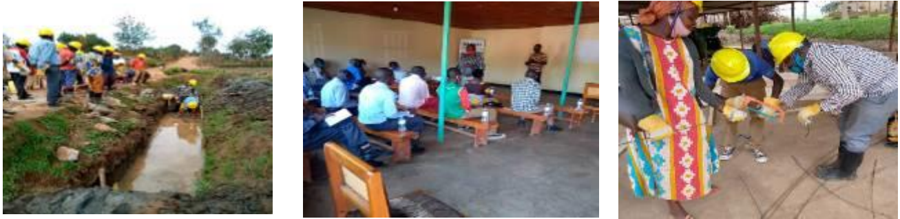
Photo 143. Preparation of foundation, Theoretical lecture and Preparation of reinforcement bar
