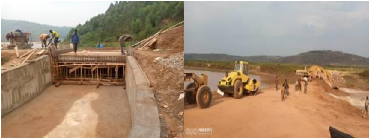
Photo 91: Dam and spillway construction at Kajevuba Dam (left) and Gashora (right)
