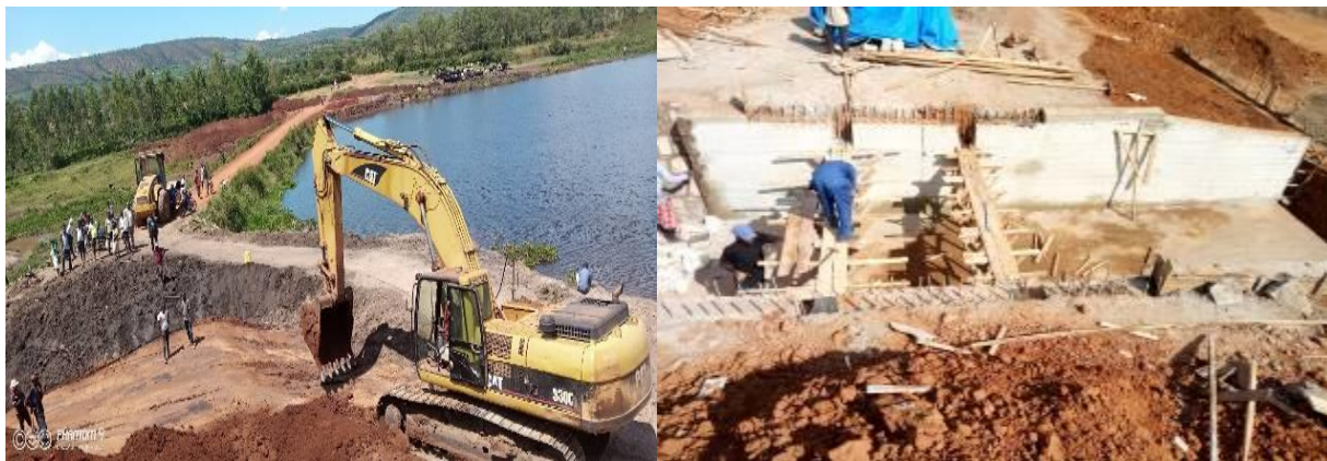
Photo 90: Bwera (left) and Rwabiharamba (right) dams under rehabilitation
