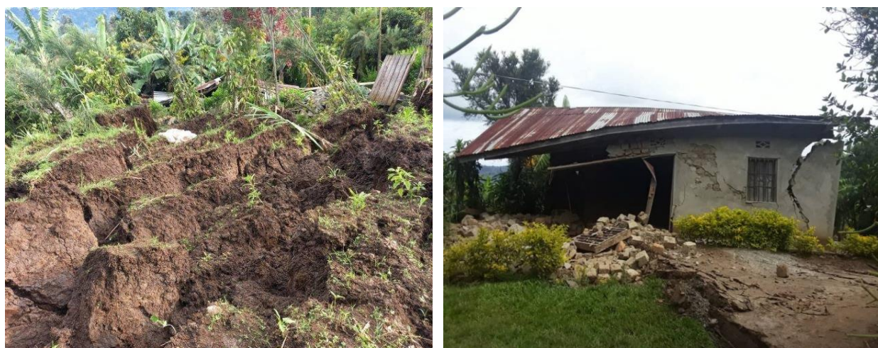
Figure 2: Landslide damage in Nyamasheke district, Rwanda, May 2021 – Photo: District of Nyamasheke
